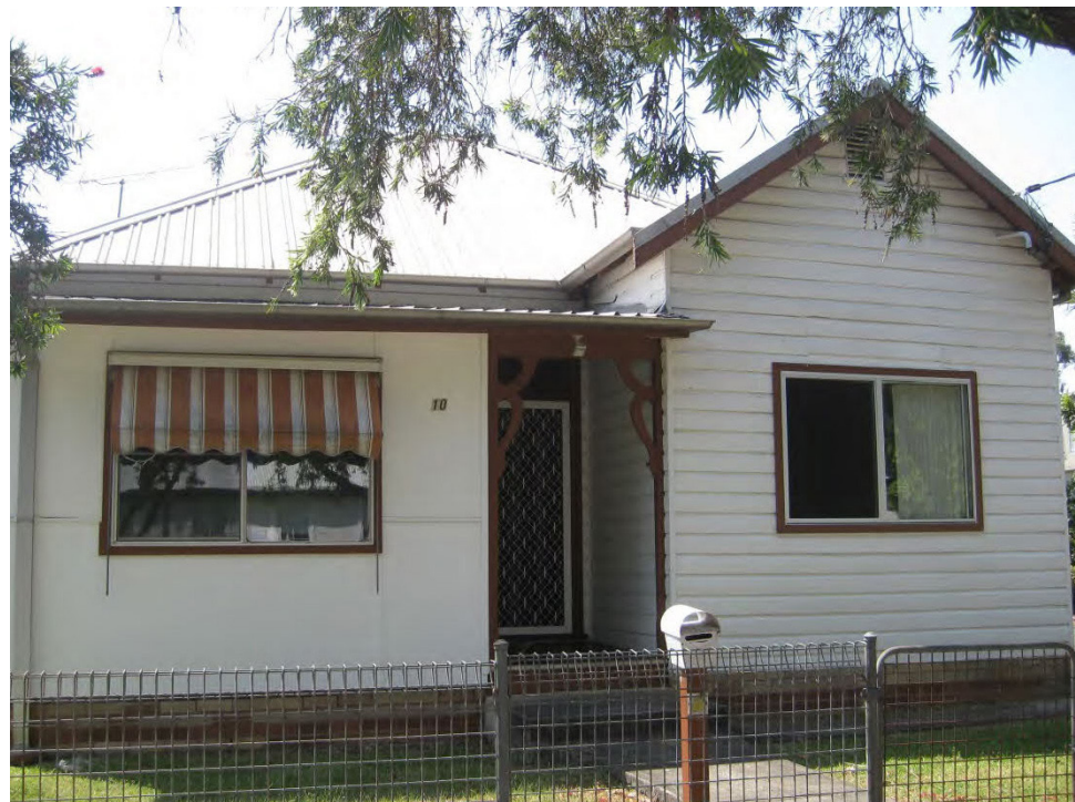
Photo 2: View of 10 Merton Street.
