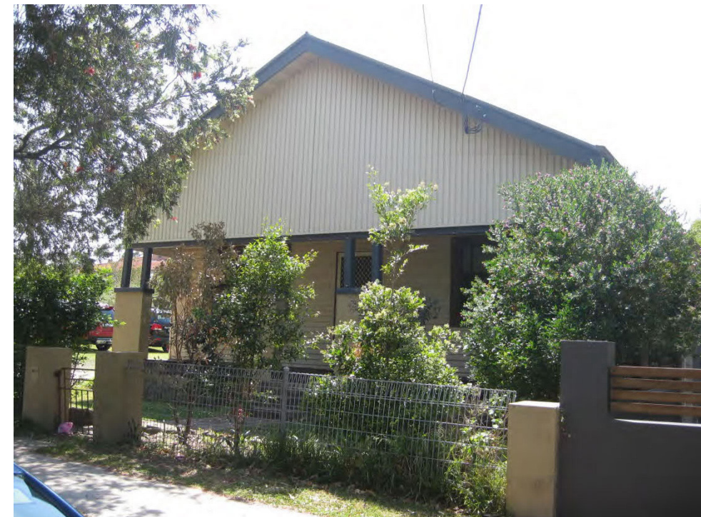
Photo 3: View of 14 Merton Street.
